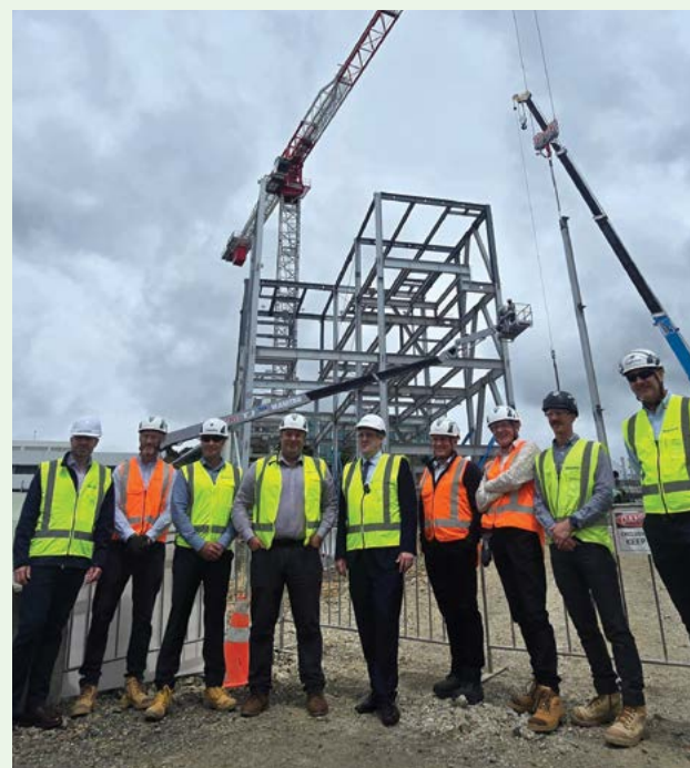
Ministers Chris Bishop and Andrew Hoggard recently toured the site of the new Plant Health and Environment Laboratory in Auckland
